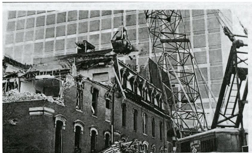
Figure 28. Demolition of Building C.
