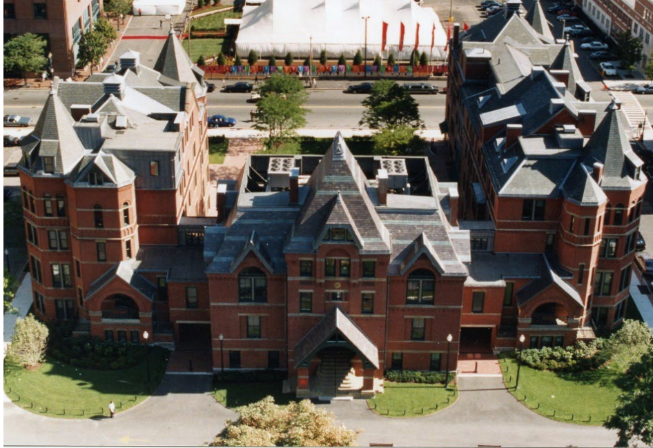
Figure 3. The Talbot Building in early 2000 before construction of the parking garage. Figures 2 and 3 were taken from the top of the Instructional Building prior to construction of the garage on Albany Street, as you can see in the background.
