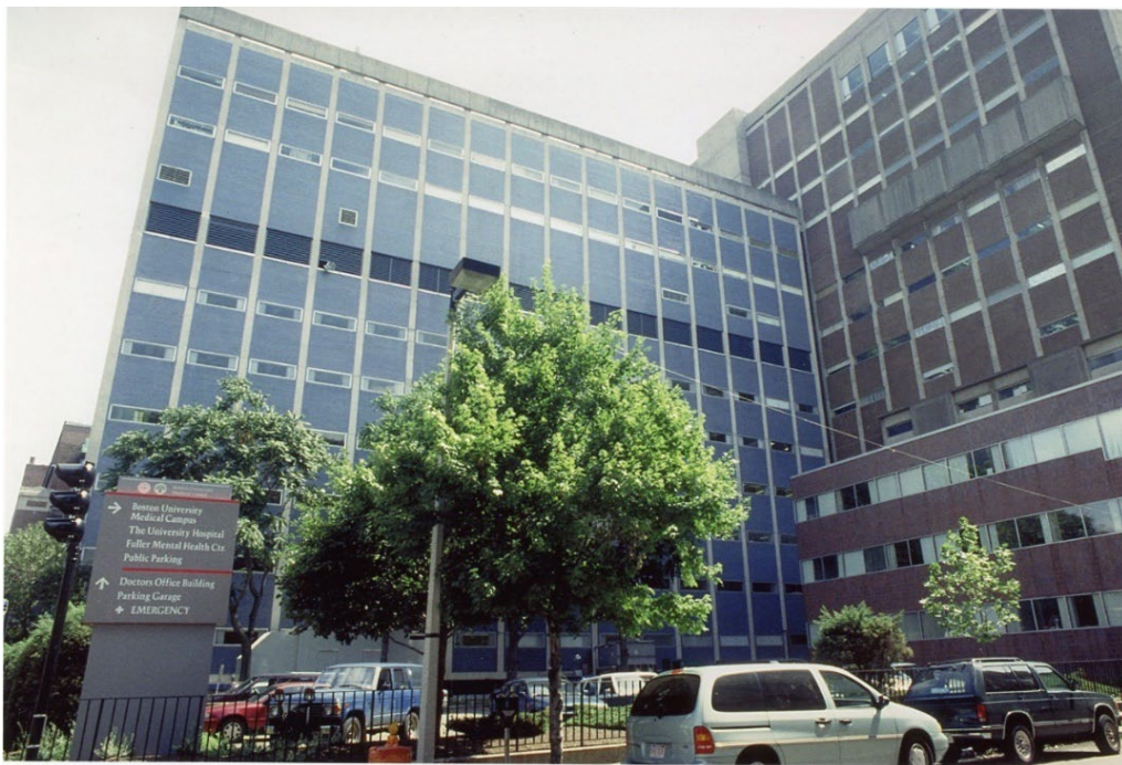
Figure 26. The “Blue Building” and parking lot on the same location in 1998.
